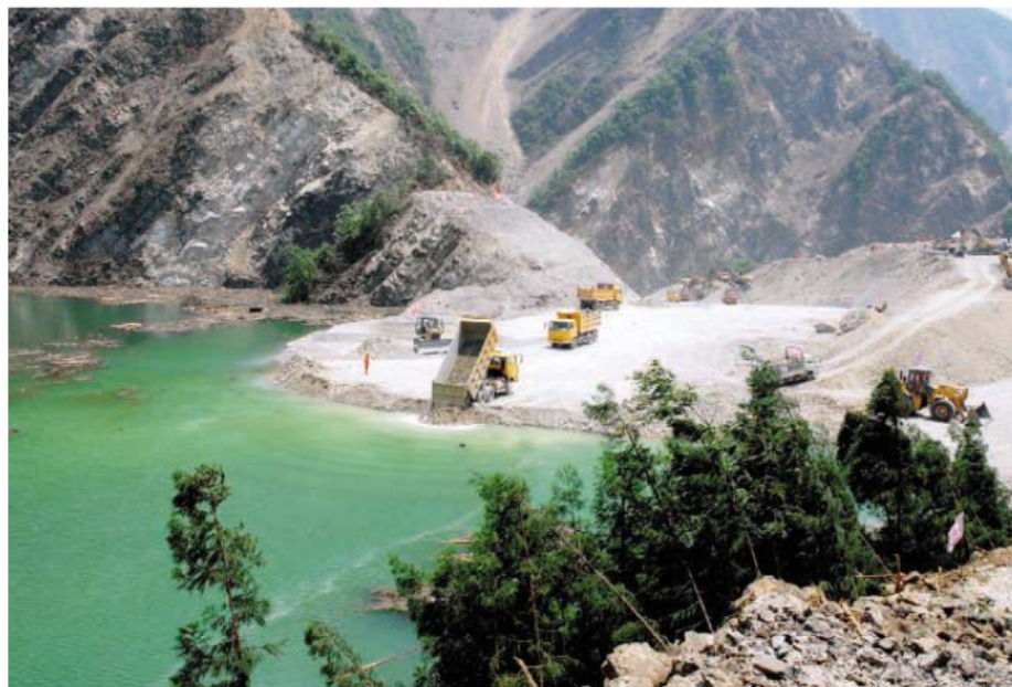
Rough-hewn floodgate. Workers sculpt a channel through debris blocking the Chaping River.
